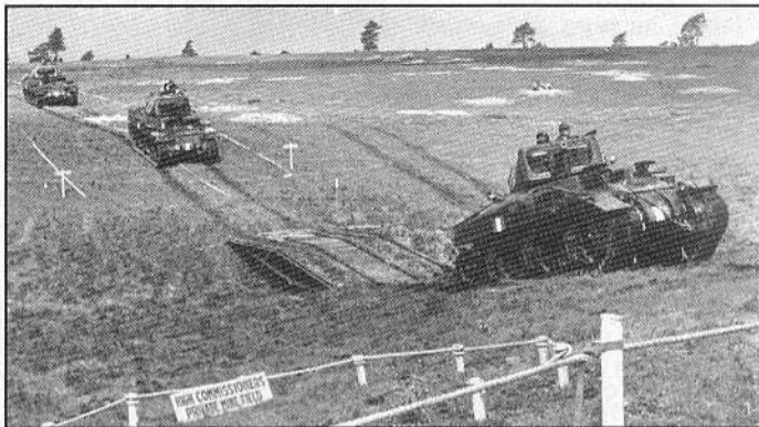
Ram II's of the 5th Cdn. Armd. Div. cross a small box girder bridge in England, May 1943. (NAC PA 192267)
